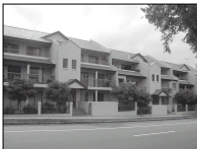
Break-up horizontal emphasis of the eaves line and roofline by inserting parapet features
